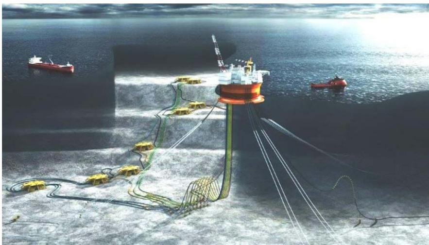
Figure 1—General view of the platform with facilities for the storage of oil - a caisson.
